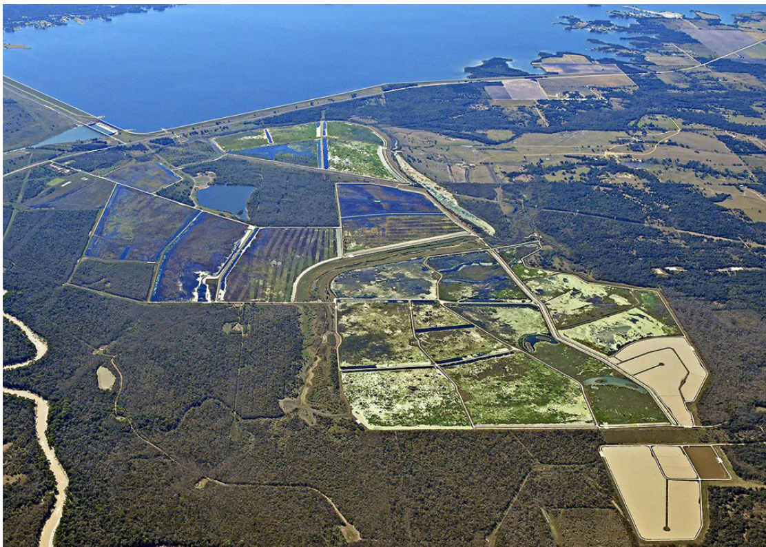
The George W. Shannon Wetlands consist of ponds and wetlands that provide habitat and recreation while treating water prior to reuse. The 2,200-acre wetlands were built as a joint effort with the Tarrant Regional Water District and the Texas Parks and Wildlife Department. Photo credit: Tarrant Regional Water District
