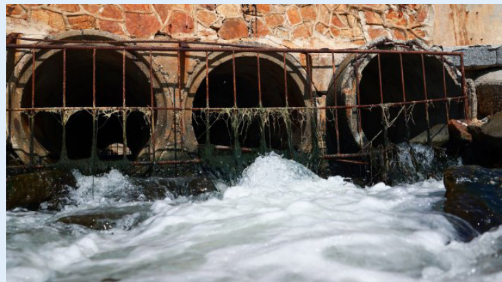
CSOs occur when the flow of wastewater and stormwater overwhelm a combined sewer system.
